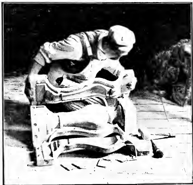
Fig. 135—Stripping the Mold from the Concrete Cast
